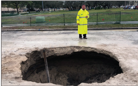
Top: Original depression that began underneath a truck on USF Magnolia Drive.
